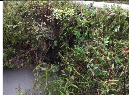
Photo 2: East Road culvert outlet.
