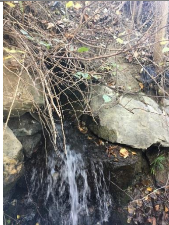
Photo 1: Murphy Hill Road culvert outlet.
