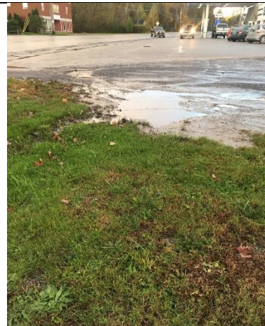
Photo 2: Impervious areas draining to the outfall and open space where a BMP could be installed.
