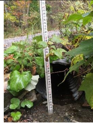
Photo 2: Potter Montgomery Road culvert inlet.
