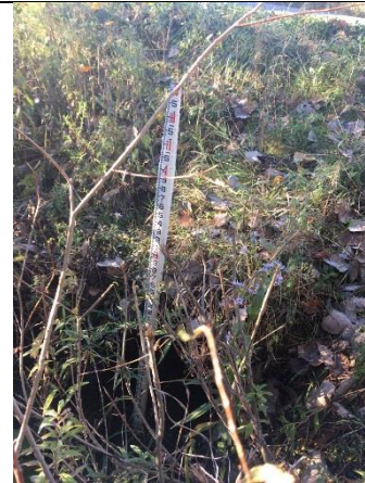
Photo 2: Murphy Hill Road culvert inlet.
