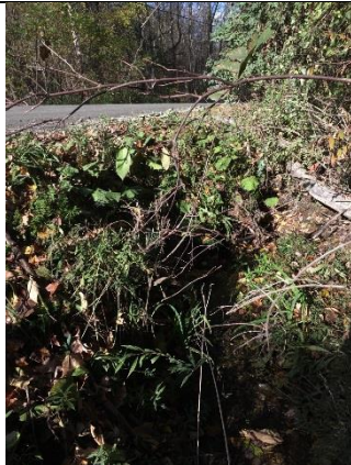
Photo 1: Murphy Hill Road culvert inlet.
