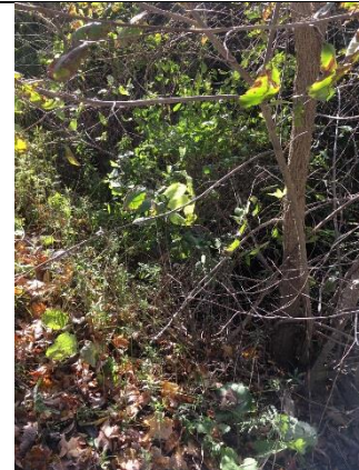
Photo 2: Murphy Hill Road culvert outlet.
