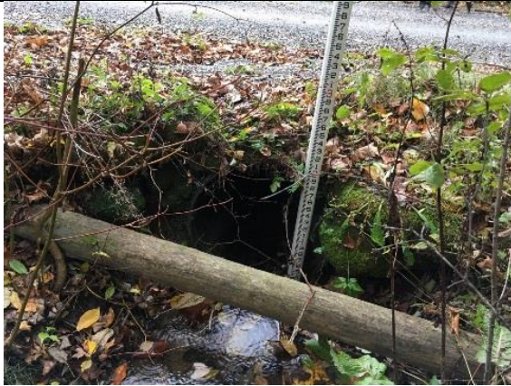
Photo 1: Potter Montgomery Road culvert outlet.
