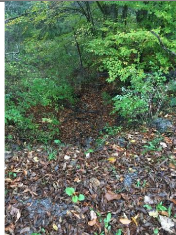
Photo 2: Eroded conveyance south of the road.
