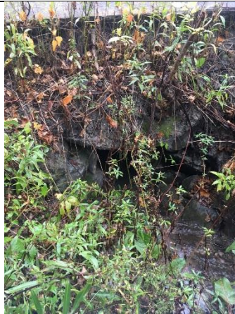
Photo 1: East Road culvert inlet.
