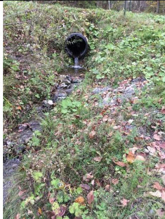
Photo 1: Harrison Road culvert outlet.
