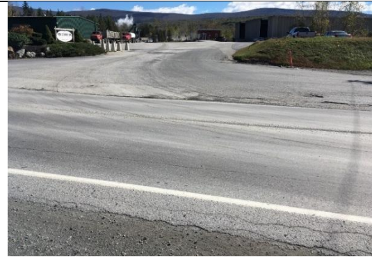
Photo 2: Route 7A and WM. E. Dailey entrance. The eastern portion of this currently drains south to stormwater infrastructure but may be rerouted.
