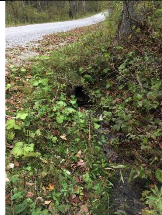
Photo 2: Harrison Road culvert inlet.
